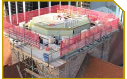
Central Tower being constructed.
